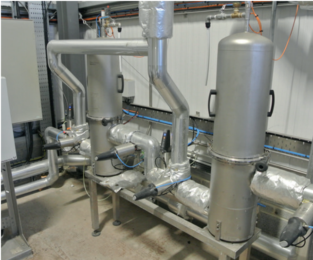
Two stainless steel PF-IG housings contain eight P-GSL N 30" cartridges each.
