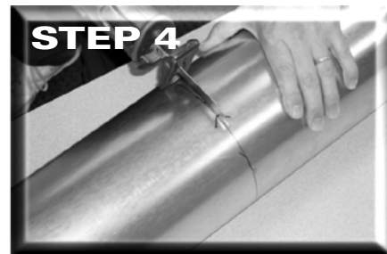
Drill access hole then cut with saw
